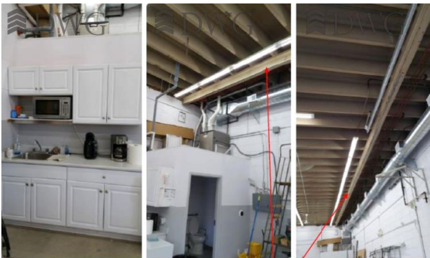
Crain rail with 2 1/2 ton capacity
